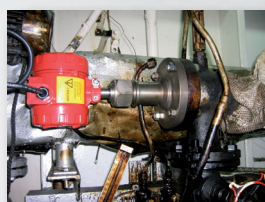
After - VISCOMASTER retrofit
