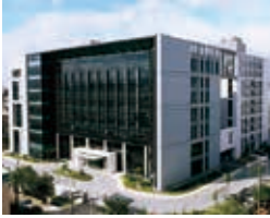
Taoyuan Technology Center (Green Building)
