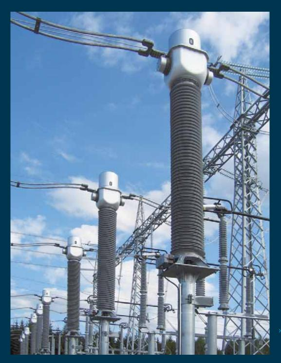
420 kV Current transformers with gray silicone rubber insulator. Statnett (Norway).
