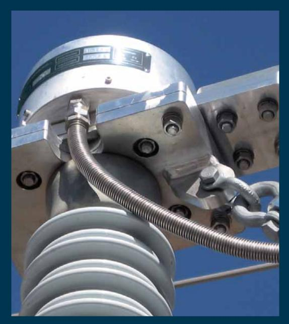
Optical current transformer SDO OCT.
